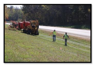
SwiftCurrent Connect construction of Phase 1 is nearly complete and Phase 2 construction has begun. Phase 3 construction is anticipated to begin next year. The fiber-optic cable follows the PPCS electric infrastructure; the cable has aerial installation where there is overhead electric service and is buried where there is underground electric service.
